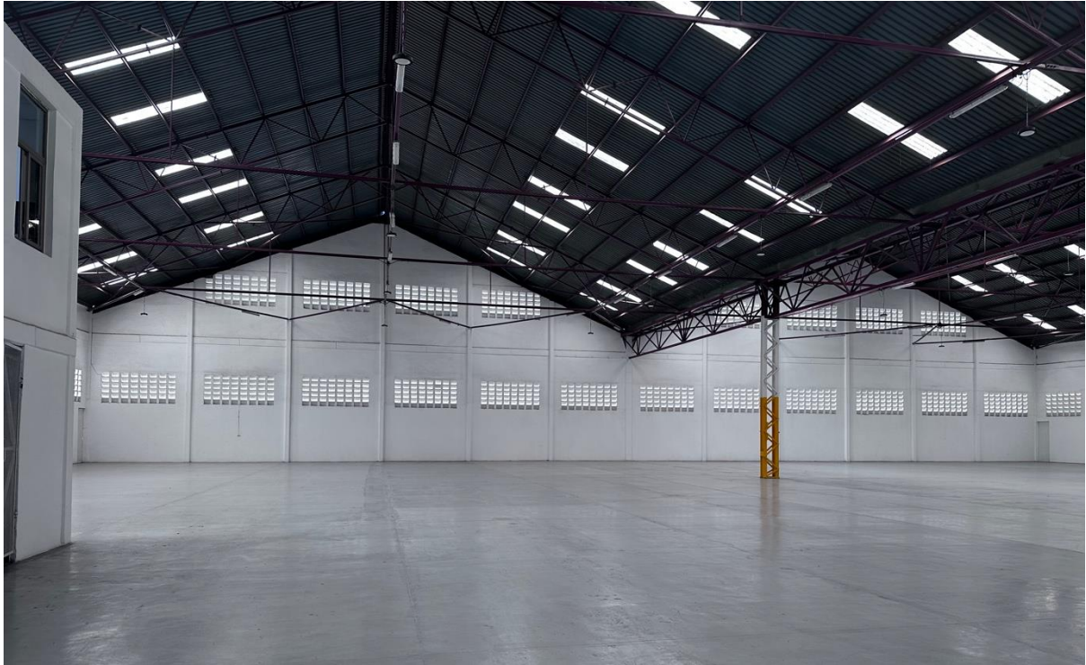
Photo 0-1 Renovated Warehouse Space at KBI
